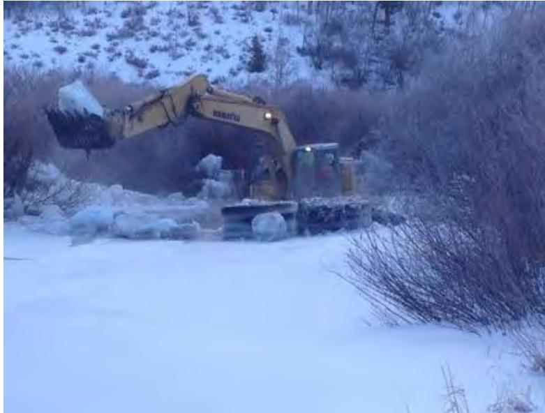
*Figure 13. This photo shows an excavator clearing massive, stratified, apparently dense ice accumulations from Flat Creek. The photo location, date, and photographer are not known.*
