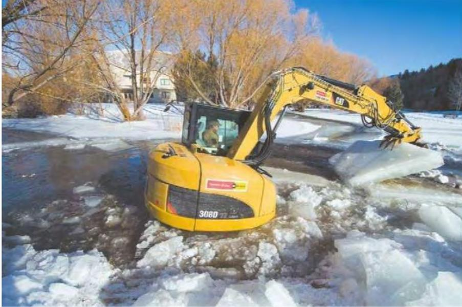
Figure 16. An excavator is shown here clearing an ice accumulation from Flat Creek at Garaman Park in early 2011.
