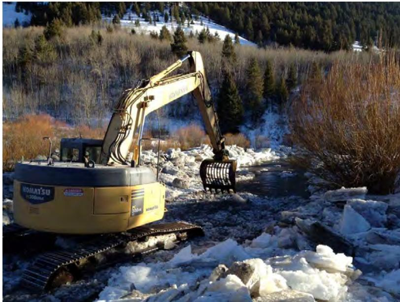
*Figure 12. This photo shows an excavator clearing ice from the creek during mid-January, 2018. The location of this photo is not known. This photo implies that the offending ice jam was not a simple ice dam that was readily cleared. Instead, it looks like many yards of the creek channel had to be cleared of ice. This image is from the Jackson Hole Underground website (<http://www.jhunderground.com/tag/flat-creek/>).*
