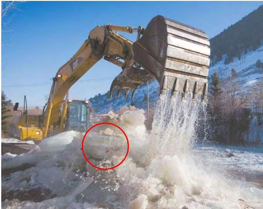
Figure 17. The excavator here is clearing ice out from Flat Creek near Garaman Park in January 2011 to relieve the risk of ice-induced flooding. The ice in the red circle appears to be a piece of merged anchor ice and border ice about 3 feet thick, which choked the creek channel.
